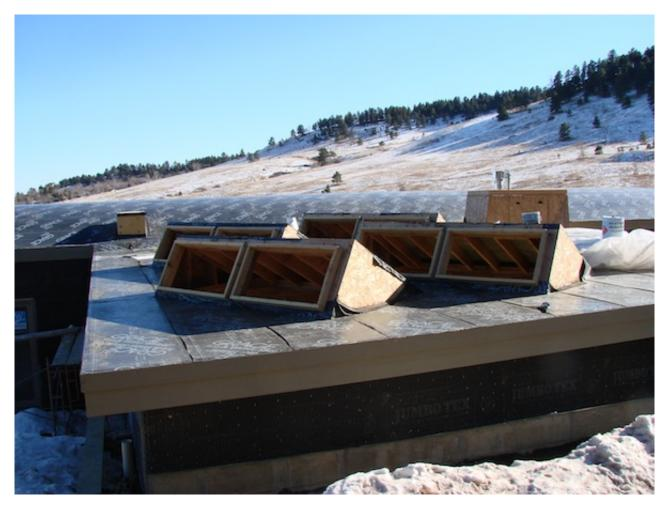
Underlayment provides temporary protection of the building interior and the roof deck before the roof-covering material is installed.
